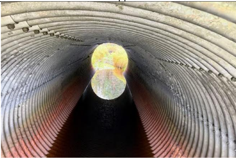
Barrel Looking West
