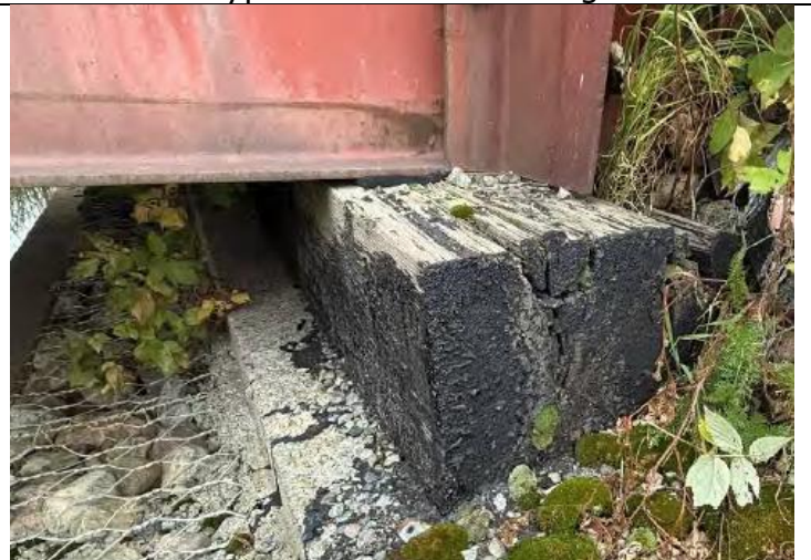
Bearing Timber - SE
